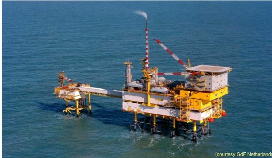
Figure 2. The K12-B offshore platform in the North Sea where CO<sub>2</sub> is injected into a sandstone formation containing natural gas. Source: [co2geonet.com](http://co2geonet.com)
