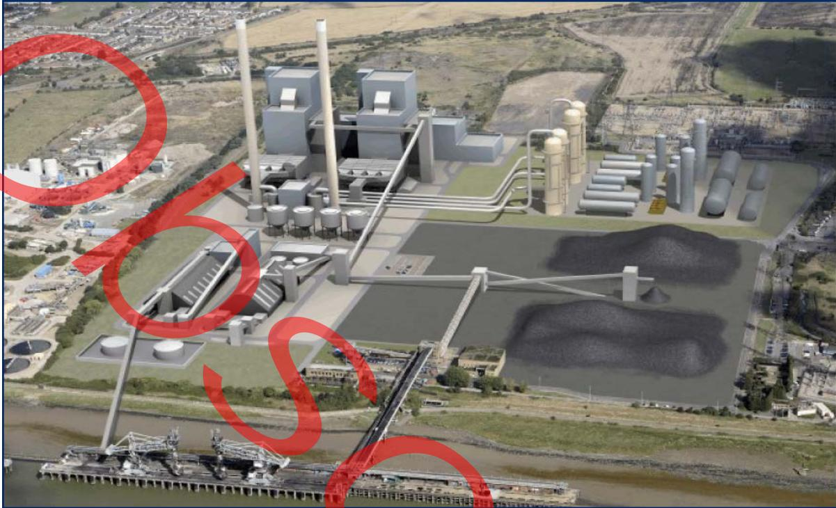
Figure 3. 2x800 MW UK coal-fired power station with capture — shown behind the coal stockpiles (sourced from Imperial College, London and RWE Group)
